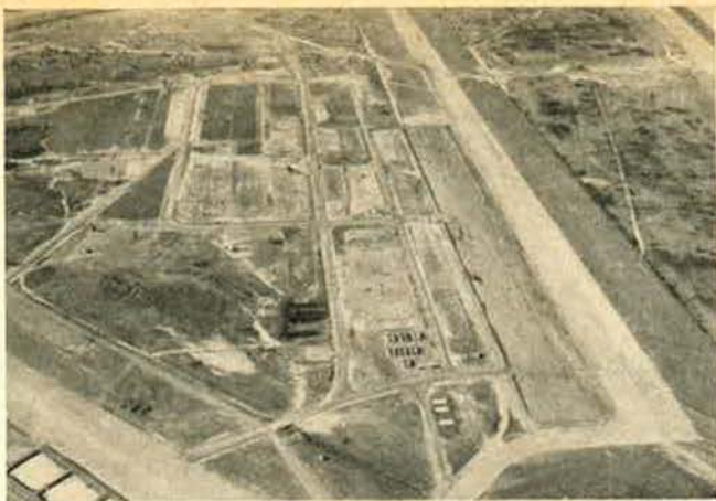
North Field, S.C., the austere site of TAC's demonstration of a new concept in tactical airpower—bare basing. The operation—called Coronet Bare—proved out the theory that a fully operational airfield can be set up from airlifted, especially designed equipment within hours.
