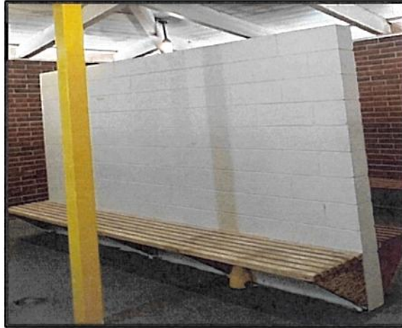
Figure 6.7: Partition Wall Prior to Mishap (Tab Z-9)
