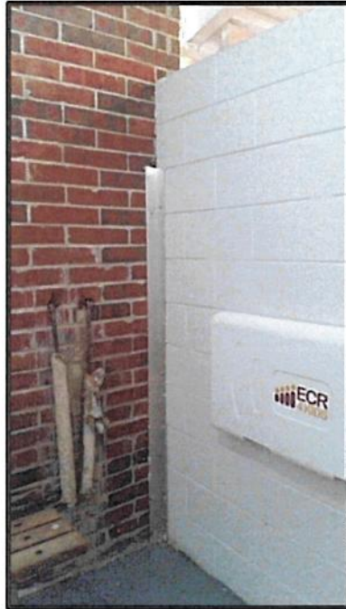
Figure 5.1: Emergency Repair to Block Wall in Women’s Restroom (Tab Z-13)
