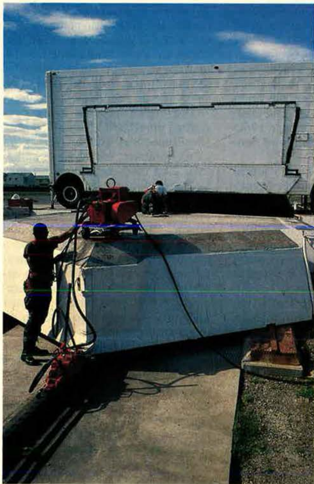
Training plays an important role in the lives of both maintainers and crews. Here, Sgt. Bill Matthews (left) and Amn. Jonathan Wood (right) train topside at Malmstrom's T-9 facility. The 110-ton blast door covering the top of the silo must be closed with a hydraulic unit known as a "pipe pusher" that moves the door three inches at a time.
