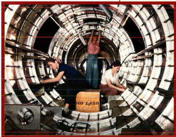
Millions of “Rosie the Riveters” entered the defense manufacturing industry. Here, women install fixtures and assemblies to a tall fuselage section of a B-17 at the Douglas Aircraft plant in Long Beach, Calif.
