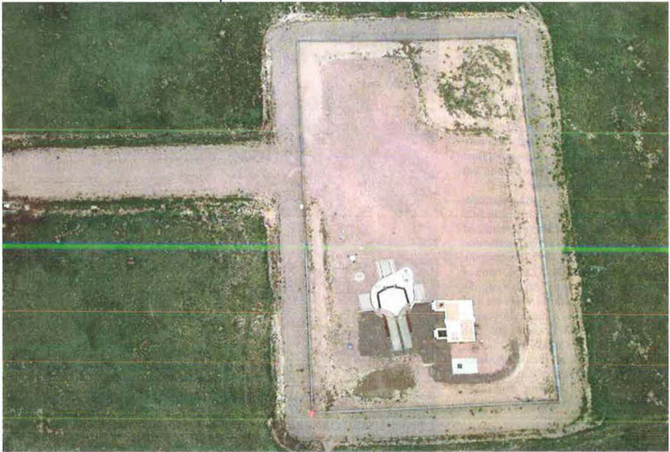
An overhead view of a Minuteman III launch facility shows the launcher door, access hatches, and some security features.
