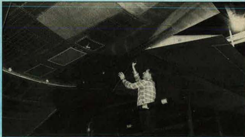
A Lockheed-Georgia Co. employee attaches a prototype "afterbody strake" underneath the empennage of a C-130 aircraft. The Air Force plans to retrofit its fleet of C-130B, E, and H models with the strakes.
