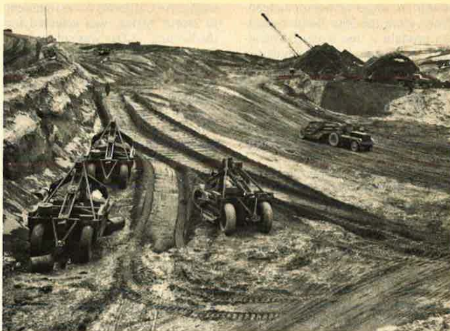
American troops landed on Amchitka in January 1943. A month later, fighters were operating from the new airstrip, and by March medium and heavy bombers were striking Kiska. Here trucks haul sand for runway foundations. The Japanese never were able to complete runways at Kiska and Attu.
