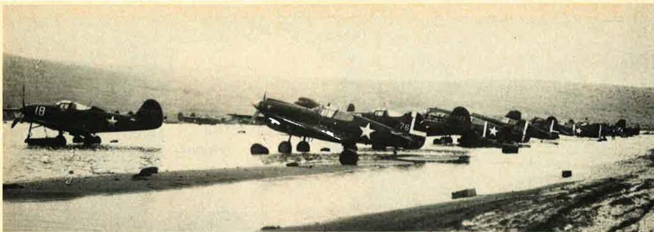
The flight line at Adak was typical of conditions at Aleutian bases during most of the campaign. P-39 Airacobras and P-40 Warhawks are among the fighters on the hardstand of this hastily built airstrip.
