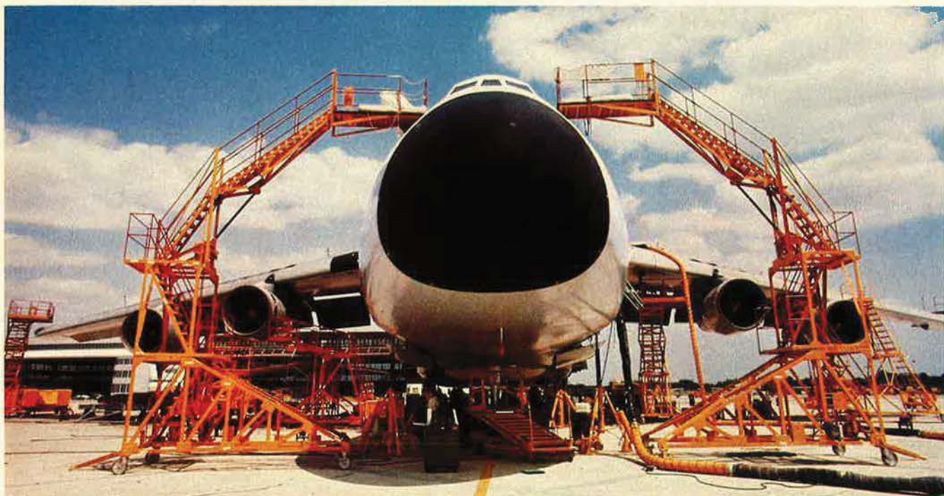
A C-5 gets programmed depot maintenance (PDM) at San Antonio Air Logistics Center. AFLC does slightly more than half of the PDM work load at its own depots and contracts out the remainder.
