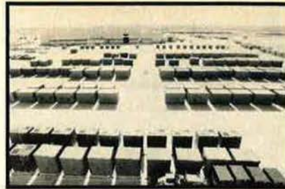
ABOVE: Rows of pallets stand sentinel at the 4449th Mobility Support Squadron, Holloman AFB, N. M. These are expandable into every type of structure required for the operation of a complete tactical air base in a remote area. They have been designed to mesh with MAC transport loading and tie-down systems. LEFT: Hard-wall, temperature-controlled shelter being erected from palletized form.
