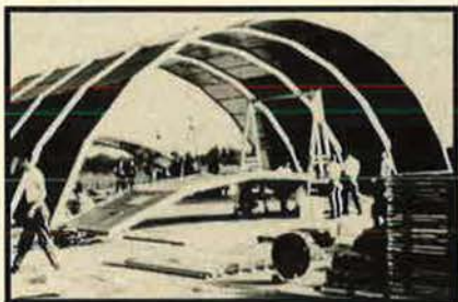
TOP: Expandable housing has been designed for strength and light weight in air-mobility role. ABOVE: Aircraft hangar, when erected, will permit entry from either end. Equipped with telephone and power outlets, it is large enough to service two F-15s or F-4s simultaneously.
