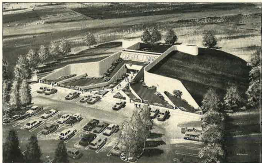
An earth-sheltered home for SAC's tanker alert crews at Fairchild AFB, Wash., is the winner of an Air Force "Design Excellence" award. The 15,000-square-foot, one-story building is situated for immediate access to tanker planes. The earth-shelter design improves security, reduces intrusion of jet noise, and is one element in the facility's energy-saving design. The facility may become a prototype for SAC bases.
