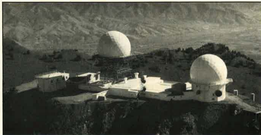
AFCC people often find their homes on remote mountaintops. These domes are typical of those used for high-frequency radio and tropospheric scatter systems.
