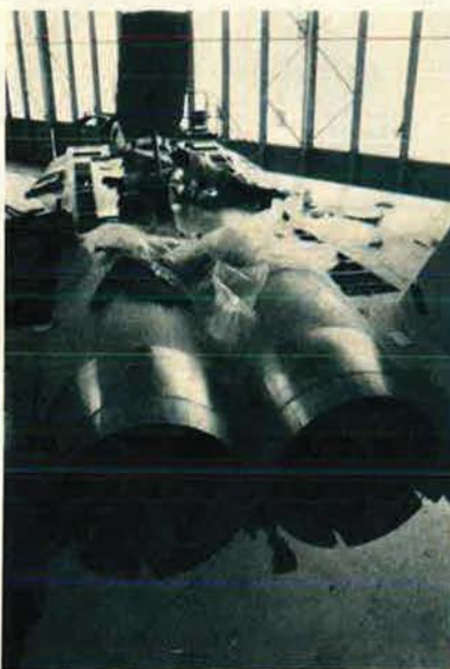
Civilian maintenance specialists on the Warner Robins ALC Speed Line perform an F-15 fuselage fuel tank modification. Three shifts operate the Speed Line around the clock.
