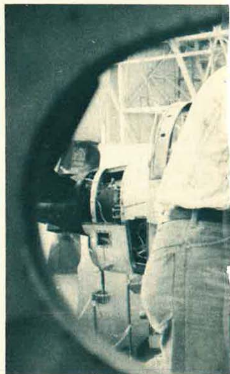
In the Warner Robins depot maintenance program, civilian repair specialist Bobby Greene works on the engine truss mount of a C-130 transport.
