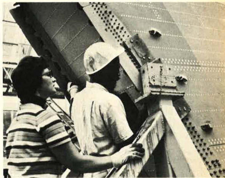
Fabrication of Boeing's 747 vertical fin.
