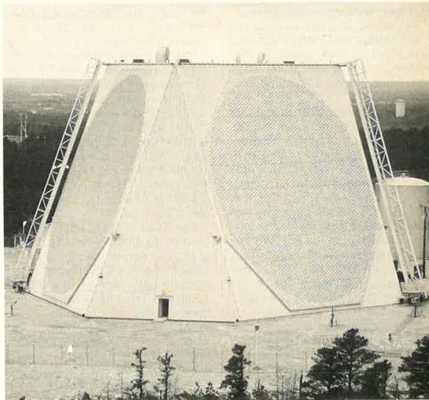
The first PAVE PAWS site, at Otis AFB, Mass., was turned over to NORAD early in 1979. The second site, at Beale AFB, Calif., will become operational late this year.
