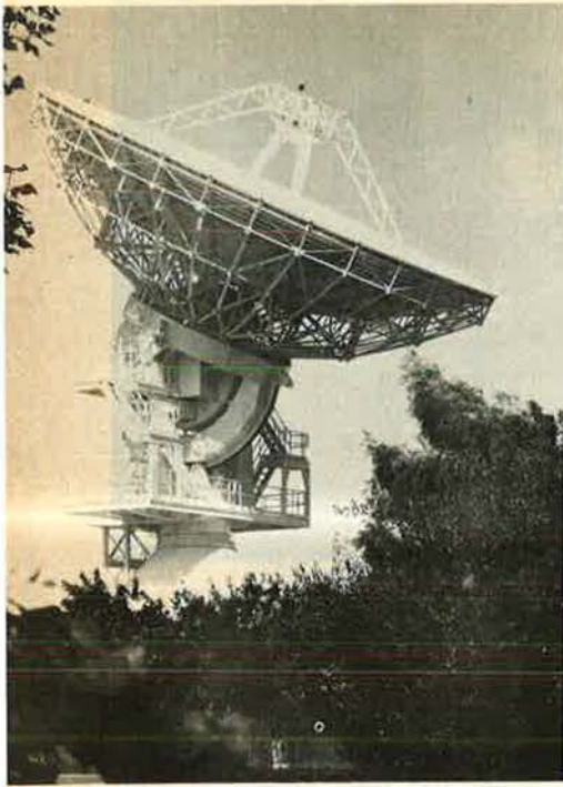
The FSC-78 satellite antenna is the heavy ground terminal for defense communications satellites.
