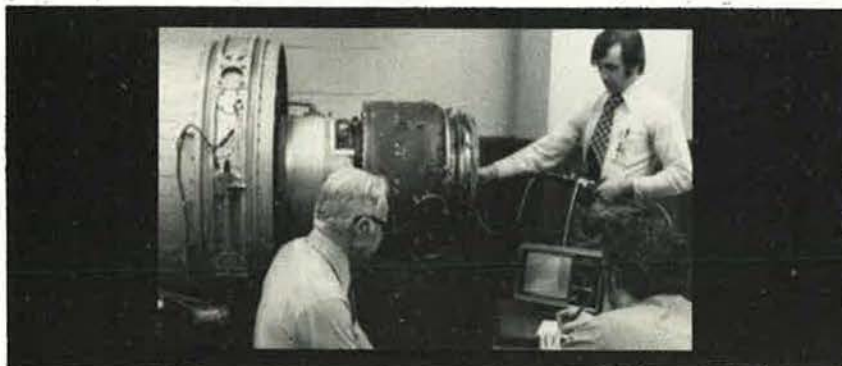
AVCO Lycoming Division engineers inspect internal areas of the ALF 502 turboprop aircraft engine. The inspection is with a flexible fiberoptic borescope.
