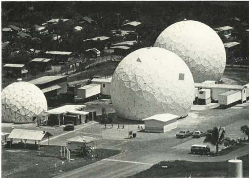
This satellite communications complex at Clark AB, Philippines, provides long-range communications for the Joint Chiefs of Staff.
