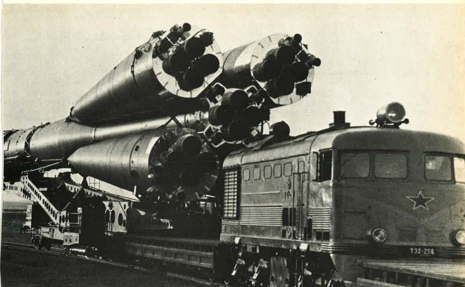
Being transported on special railway equipment is a Soyuz launcher, the central element of the Soviet Union's space program, both military and civil. With the February launch of two cosmonauts, manned flights continued into 1977.
