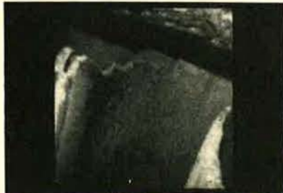
An enlargement of a photo taken in color with an Olympus flexible fiberoptic borescope, by an engineer inspecting the hot section of a gas turbine engine. The discovery might have avoided major damage and substantial tear-down and repair costs. Flexible borescope inspections pay off.
