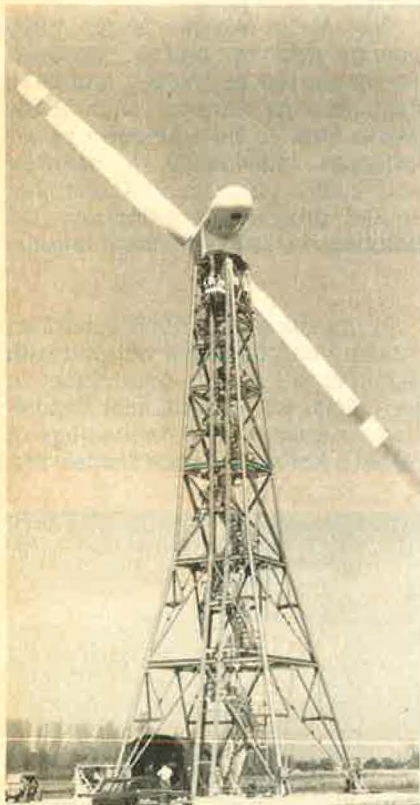
Designed to fill the electricity needs of twenty-five homes is this ERDA experimental wind energy turbine at NASA's Plumb Brook Station near Sandusky, Ohio. The huge windmill, built by Lockheed-California, is part of Project Independence—a move to reduce US reliance on foreign energy sources. Wind energy research promises bountiful returns.
