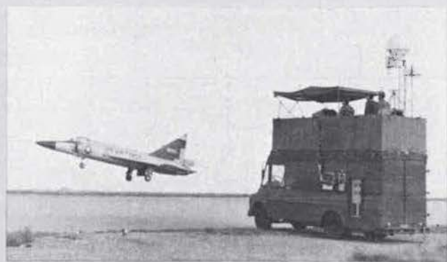
Sperry (Convair/General Dynamics) PQM-102, the first-ever fighter aircraft converted for drone duties with no provision for manned flight
