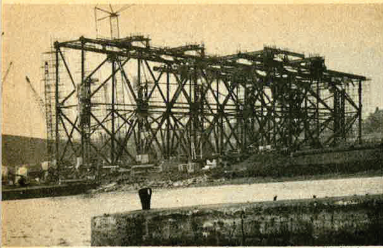
One of the UK's North Sea production platforms under construction at Methil, Scotland. Upon completion, it will be towed to a location west of Ekofisk.
