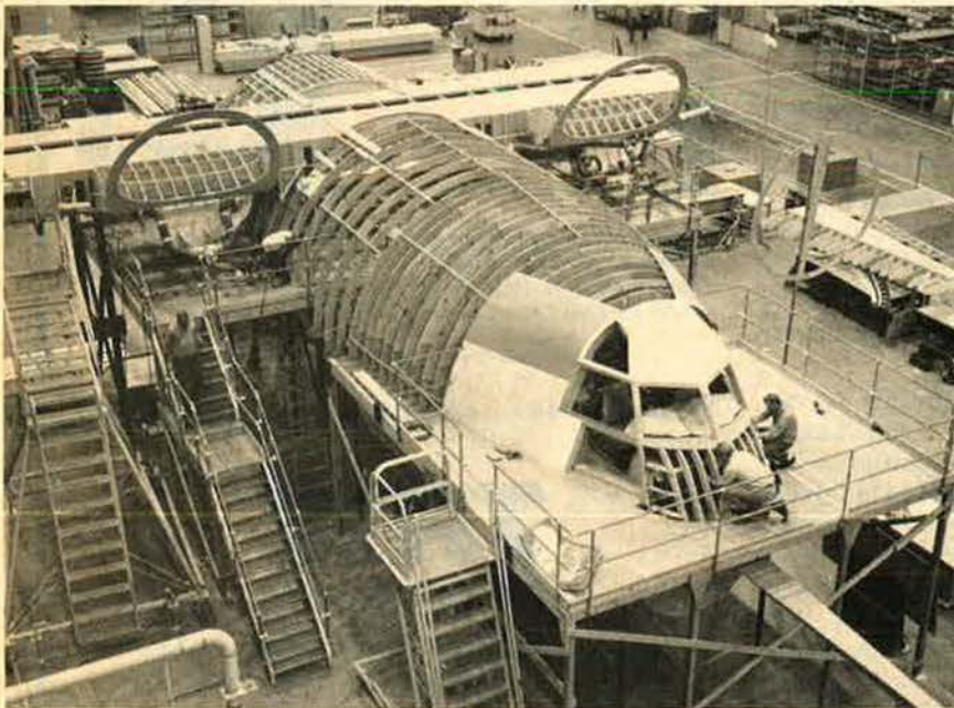
Technicians work on a full-scale, wooden mockup of the YC-14, Boeing Co.'s entrant in the Air Force's Advanced Medium STOL Transport competition. The two ovals attached to the wings' leading edges represent the aft end of engines mounted to exhaust over wing and flap surfaces—a new concept for STOL. Continued DoD funding of the AMST program is currently in question.
