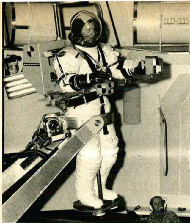
Astronaut Paul J. Weitz trains on the Maneuvering Unit Simulator at Martin Marietta Aerospace Corp. near Denver, Colo. He and fellow astronauts Conrad and Kerwin are finishing training in preparation for the first Skylab mission, set for mid-May launch (see below). The maneuvering unit is a jet-powered backpack worn over normal clothing or spacesuit.
