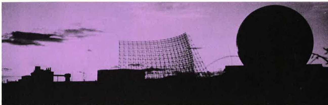
A tree and some brittle grass poking from the snow frame this Clear, Alaska, BMEWS site. Visible are tracking radar (right), detection radar screen (center), and power plant (left). Such missile detection sites provide a slender edge of fifteen minutes of warning.
