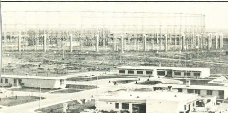
Referred to as the "Elephant Cage," this circular disposed antenna array is one antenna system employed in USAFSS communications monitoring activities.
