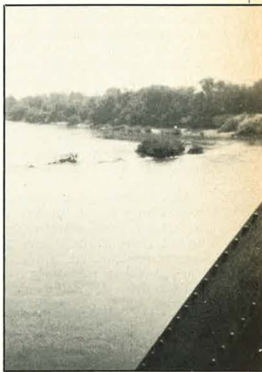
Viewed from the steel bridge in 1971, all that's left of the celebrated wooden bridge is silt and broken pilings.
