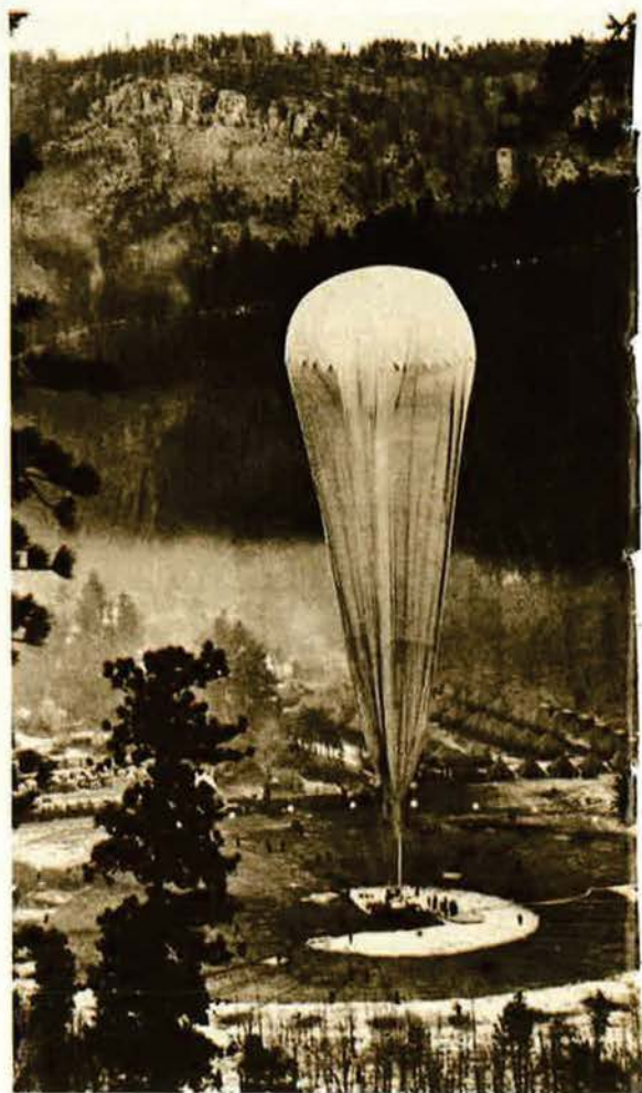
On November 11, 1935, Explorer II is readied at the Strato Bowl camp—a natural depression in the earth that served to protect the balloon from winds before launch. The record-setting flight began at 7:00 a.m.
