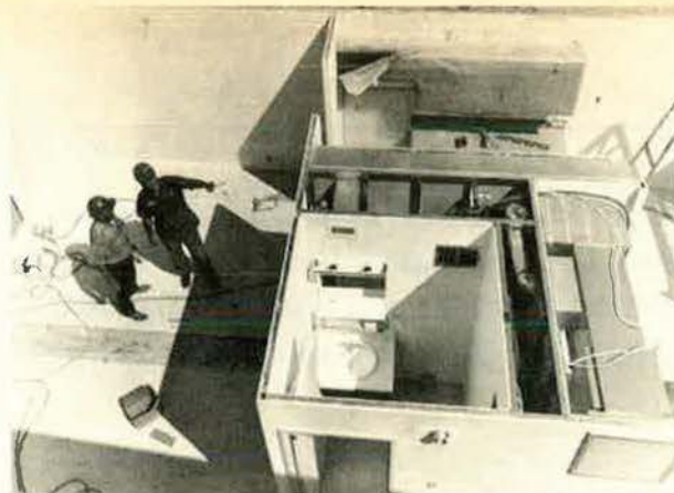
Progression from combined plaster mold/steel-frame wall panels to modules that can be erected at the site is swift under the USAF method.
