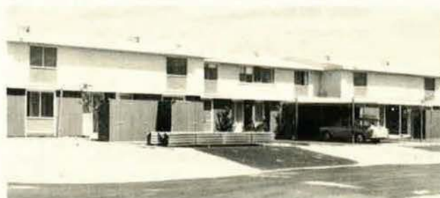
All that's needed to erect a town house at the building site is a small work force and a conventional crane. Modules, including the utility core units, leave the housing factory in finished form. Landscaping is the only remaining task before the homes can be occupied.
