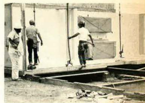
Progression from combined plaster mold/steel-frame wall panels to modules that can be erected at the site is swift under the USAF method.
