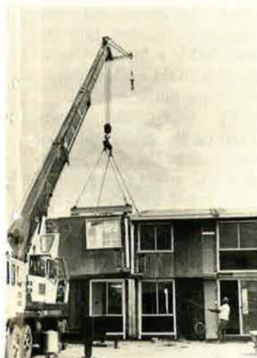
All that's needed to erect a town house at the building site is a small work force and a conventional crane. Modules, including the utility core units, leave the housing factory in finished form. Landscaping is the only remaining task before the homes can be occupied.
