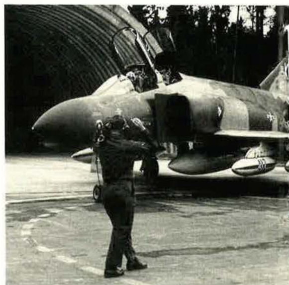
Hundreds of steel, trussless-arched shelters are being built throughout USAFE to provide protection against surprise attack on USAFE aircraft.
