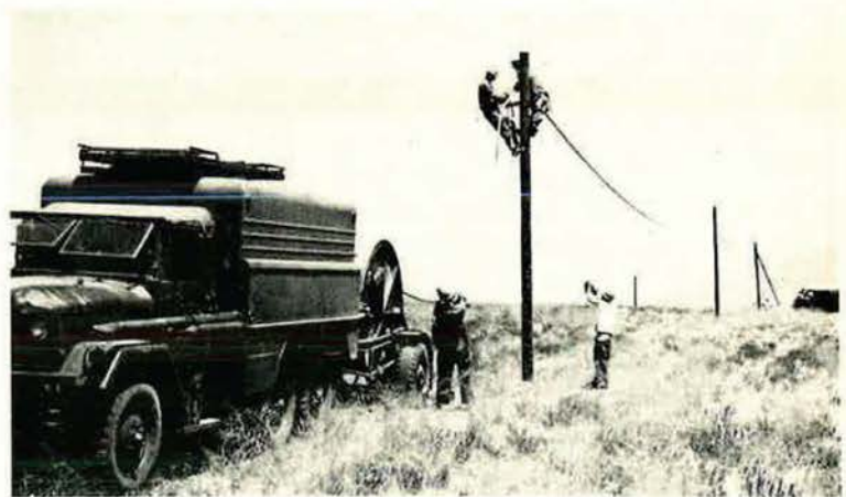
Hill AFB, Utah, is a site for training of ANG personnel in the art of stringing power lines.
