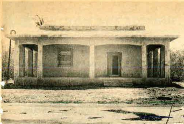
Still standing more than a quarter century later is this Japanese-constructed air operations building on Tinian.
