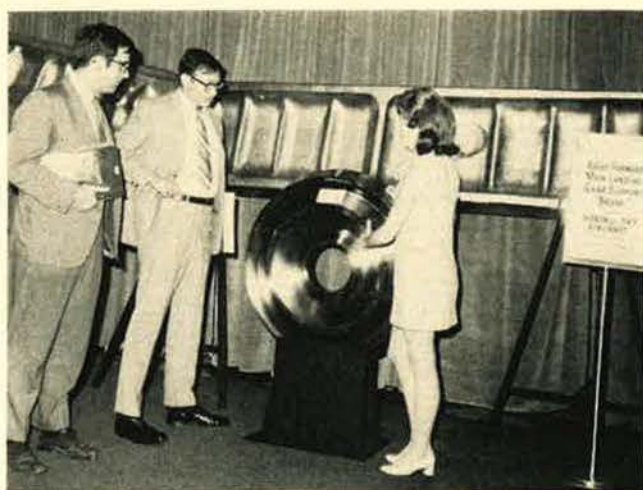
Largest titanium beam ever forged, shown by Wyman-Gordon, is made for main landing-gear support in the Boeing 747. Four beams, each weighing 4,000 pounds, go in each plane.
