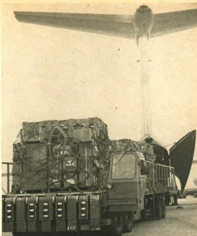
Cargo is loaded on a C-141 transport with the use of a special loader that can lift 25,000 pounds. The big aircraft, at Kelly AFB, Tex., is headed for Southeast Asia.
