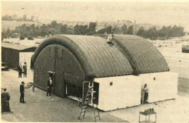
Developed for rapid deployment to any part of the world, the shelter shown above has an air-inflatable roof and walls. The Air Force Electronic Systems Division's 407L program involves the design of a whole generation of such equipment to meet USAF's requirement for quick response.
