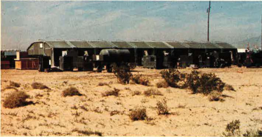
2 June, 1980 Nellis AFB...mobile buildings are ready for AIS...
