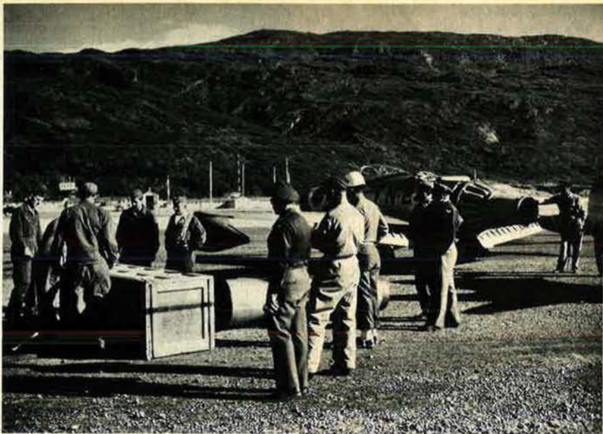
Supervising the uncrating of a tailpipe at BW-1 to replace one buckled by heat, one of the few major maintenance problems encountered during the transatlantic crossing and return.
