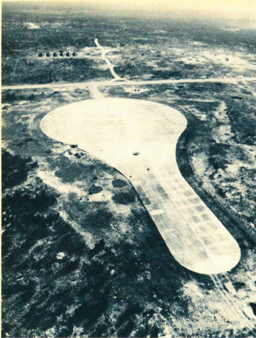
The "Ping-Pong Paddle" concrete target used for tests of foreign airfield attack munitions at Eglin AFB, Fla.
