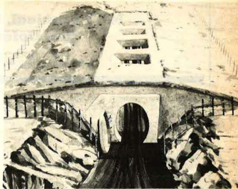
ABOVE: The most sophisticated and expensive of the MXIMPS variants is the horizontal dash. This artist's concept shows one of the twenty-three "dash" version shelters in a grid, with its ports open for inspection.
