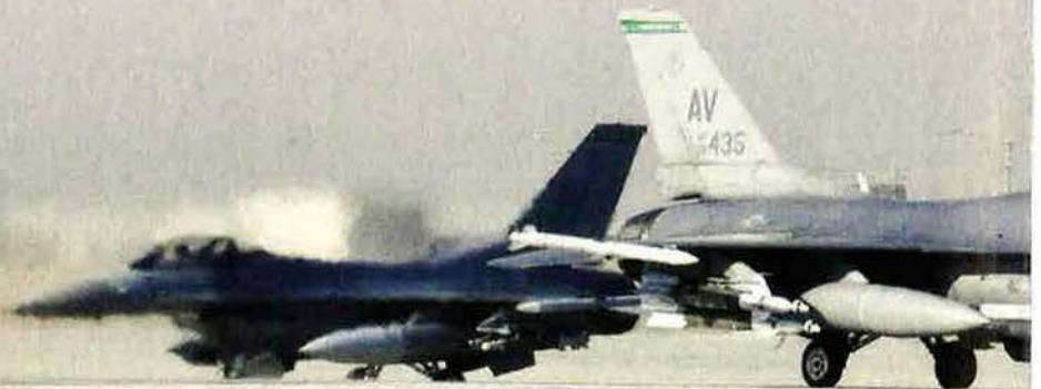
TSgt. Christopher Fitzgerald examines the runway at Bagram Airfield as rubber from the tires of jets taking off and landing is removed from the surface with foam and biodegradable solvents.
