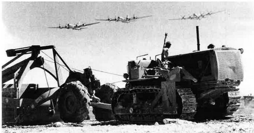
B-29s sweep low over the Marianas as a US Navy construction battalion (Seabees) builds a base. XXI Bomber Command would drop 156,000 tons of bombs operating from the chain of tiny islands.
