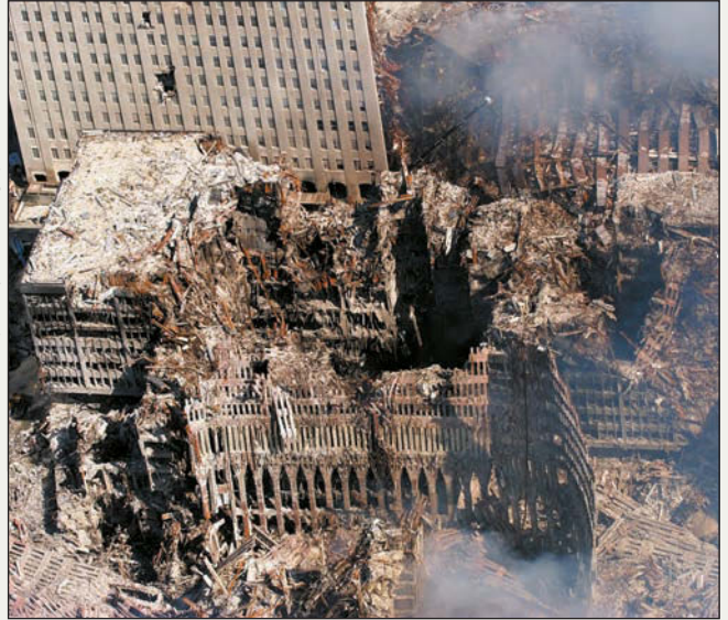
An aerial view of the damage in NYC. Scarfuto spent weeks aiding the cleanup and recovery effort.
