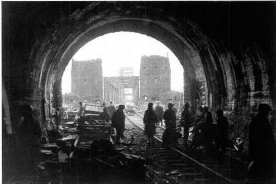
US troops and equipment move across the Ludendorff Bridge in Germany. With airpower isolating the German troops near Remagen, the Allies were able to use the bridge to cross the Rhine.
