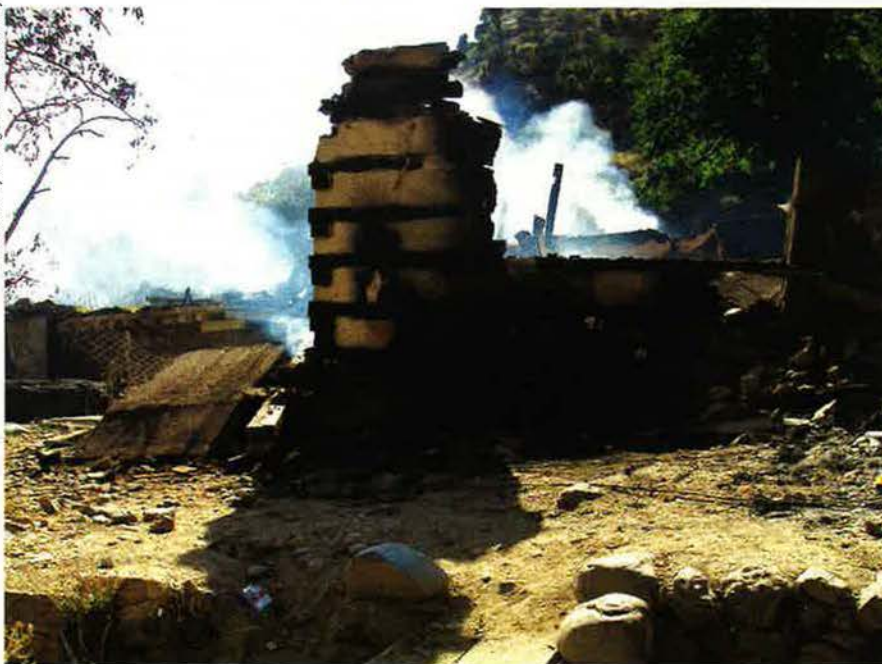
The remains of a building at COP Keating smolder after the insurgent attack. By the time of the attack, there was no longer a tactical or strategic value to holding the post.
