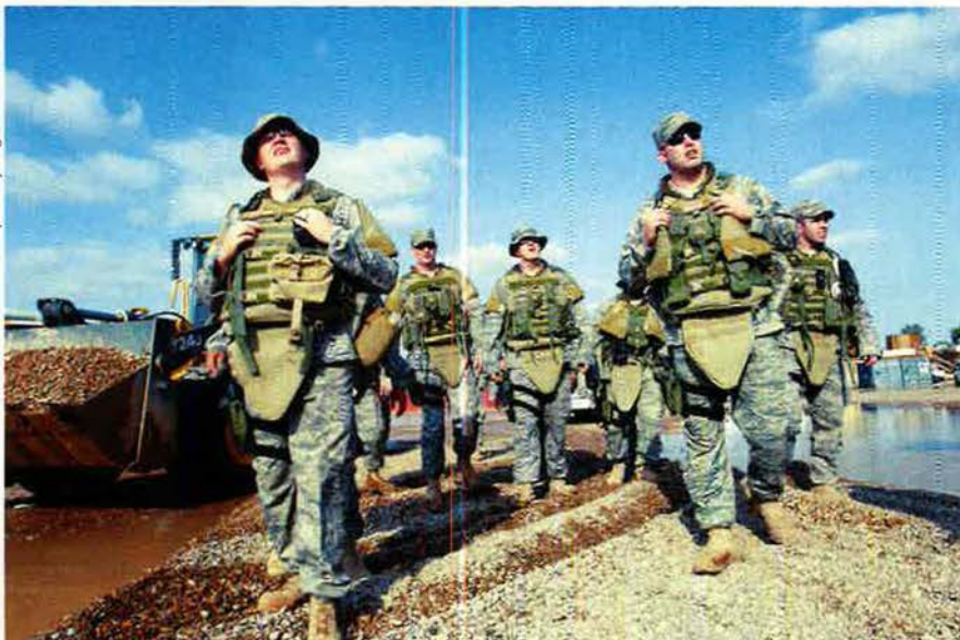
Heavily protected airmen of the 532nd Expeditionary Security Forces Squadron survey a construction site at the Balad base.
