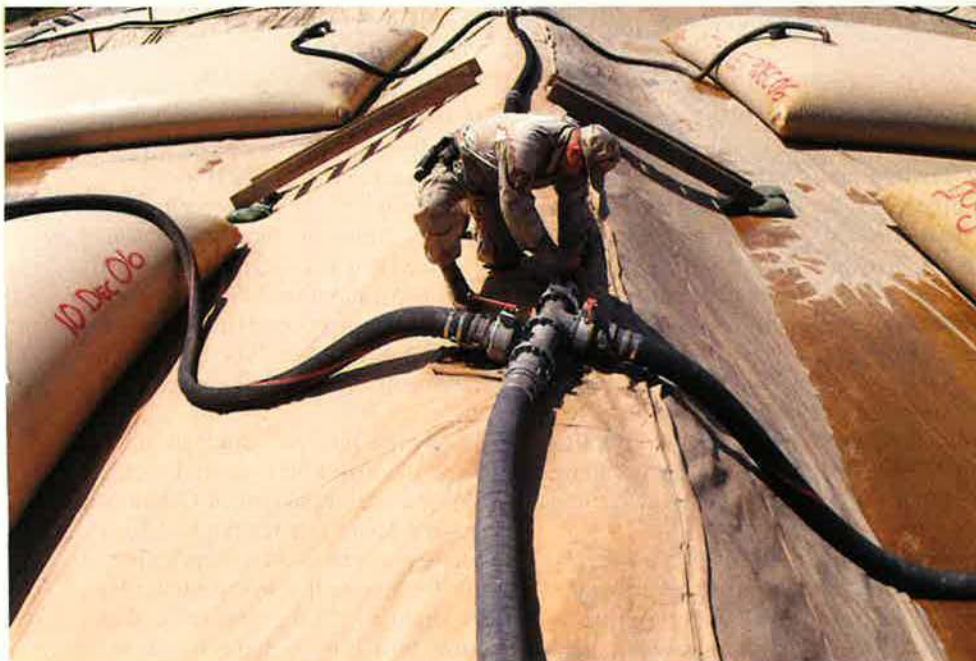
TSgt. Adam Giles closes a block valve on a 50,000-gallon JP-8 fuel bladder at Kirkuk AB, Iraq. The "bladder farm" provides fuel for five forward operating bases in addition to Army and Air Force operations at Kirkuk.
