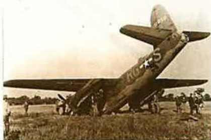
Above, this B-26 Marauder landed hard in England in September 1943 after flak had hit its landing gear lock.
