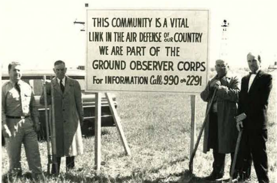
Pictured is a groundbreaking ceremony for a GOC observation post in New York state. GOC posts were constructed on top of existing buildings or on hilltops—any place with a clear, unobstructed view of the sky.
