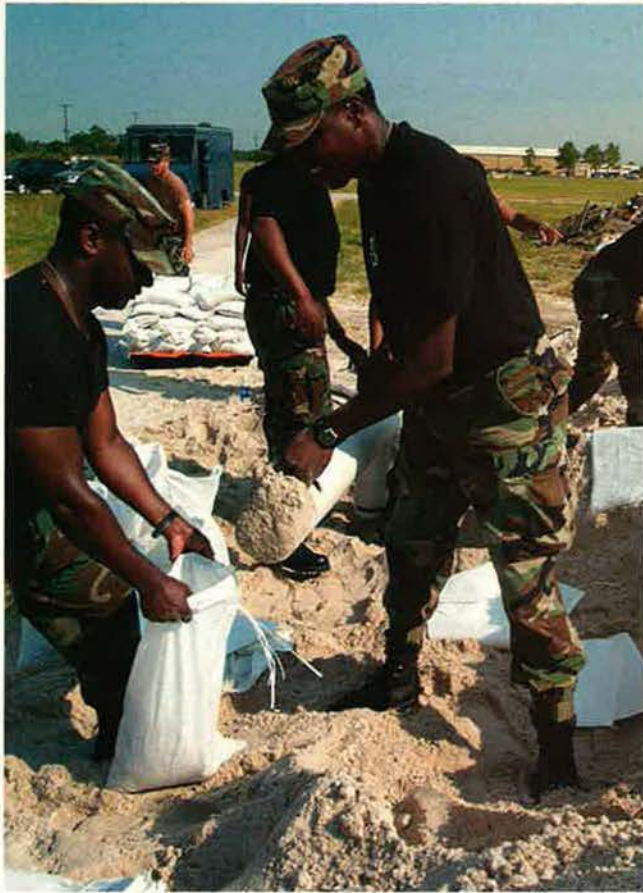
Above, airmen with ANG's 147th Fighter Wing, Ellington Field, Tex., fill sandbags to forestall water damage to base buildings from approaching Hurricane Rita. Ellington is located 10 miles southeast of Houston.
