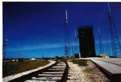
Rail lines (left and below) carry assembled rockets to their protective launch gantries. Each gantry is surrounded by four metal towers (below) that draw lightning strikes away from the assembled rocket. The photo at left was taken from the vantage of a gantry.
