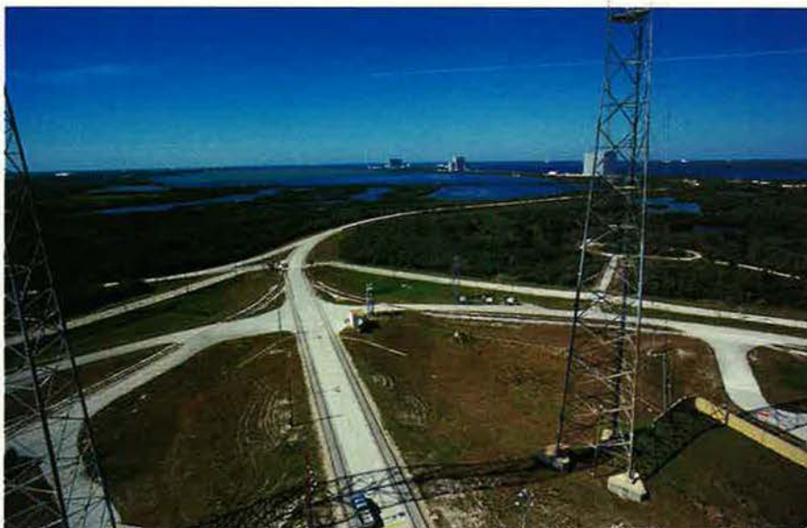
Rail lines (left and below) carry assembled rockets to their protective launch gantries. Each gantry is surrounded by four metal towers (below) that draw lightning strikes away from the assembled rocket. The photo at left was taken from the vantage of a gantry.
