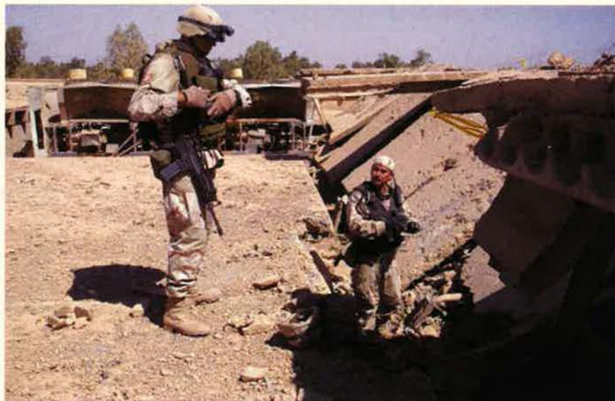
Battle damage assessment needs to be faster. Here, SSgt. Tony Newbern (left) and MSgt. Eddy Dominguez, explosive ordnance disposal technicians, find an unexploded bomb embedded in a Baghdad roof.
