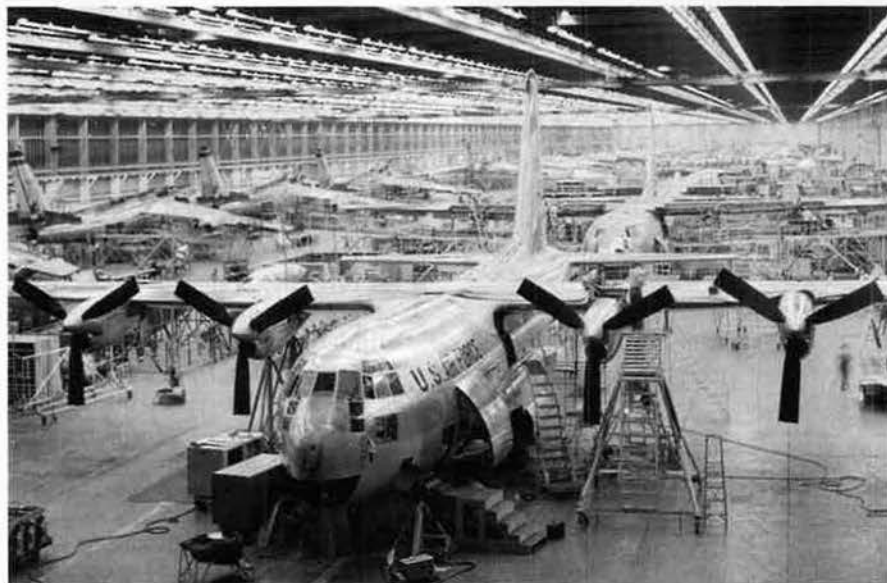
Lockheed built the prototype C-130s in Burbank, Calif., but moved production to Marietta, Ga. (above), where it is today. In 1951, B-47 production (in background) was ending.
