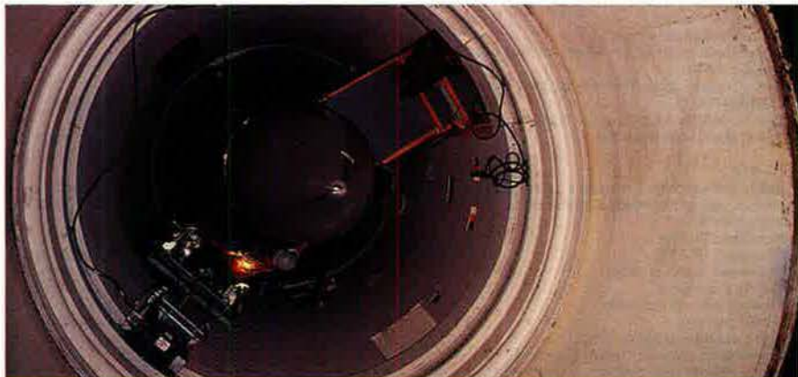
LGM-30G Minuteman III in its silo (Guy Aceto)
