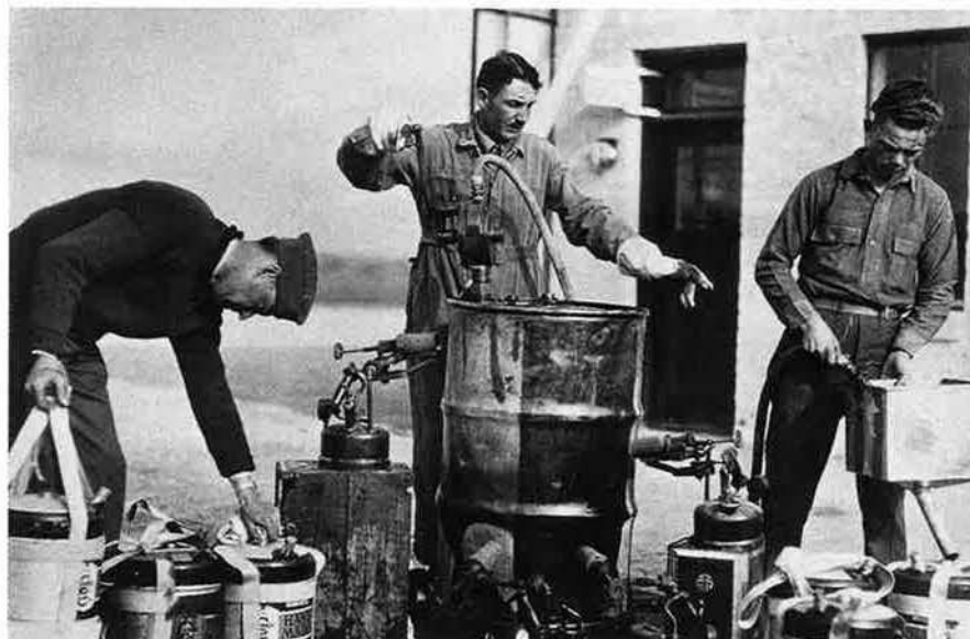
A ground crew prepares preheated oil in five-gallon cans that the refueling aircraft will lower through the hatch of Question Mark .
