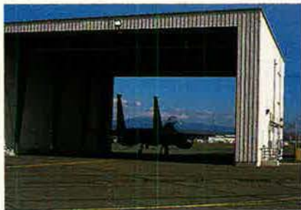
The need for more aircraft on alert to cover their area of responsibility moved up planned construction of four new alert hangars on the 142nd Fighter Wing's flight line.
